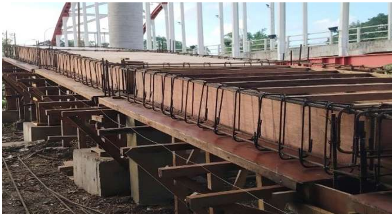
Installation of formwork and reinforcement for the bridge approach.
