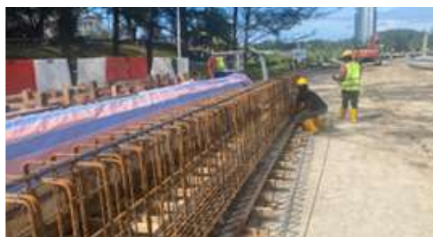
Progress of foundation works through spun pile installation
