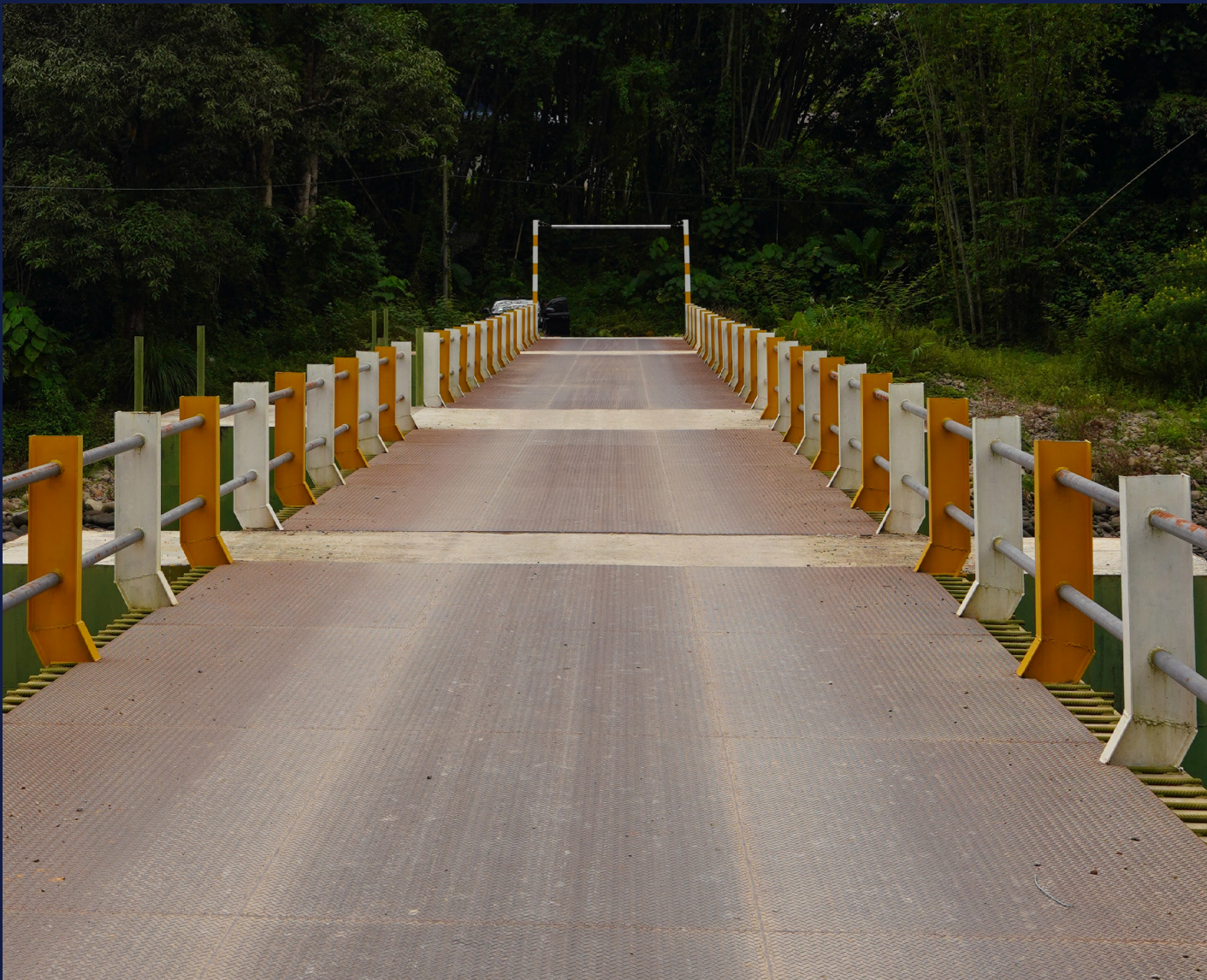
Projek Baikpulih ‘Low Level Crossing’ Kg. Poturidong Kiulu, Tamparuli
