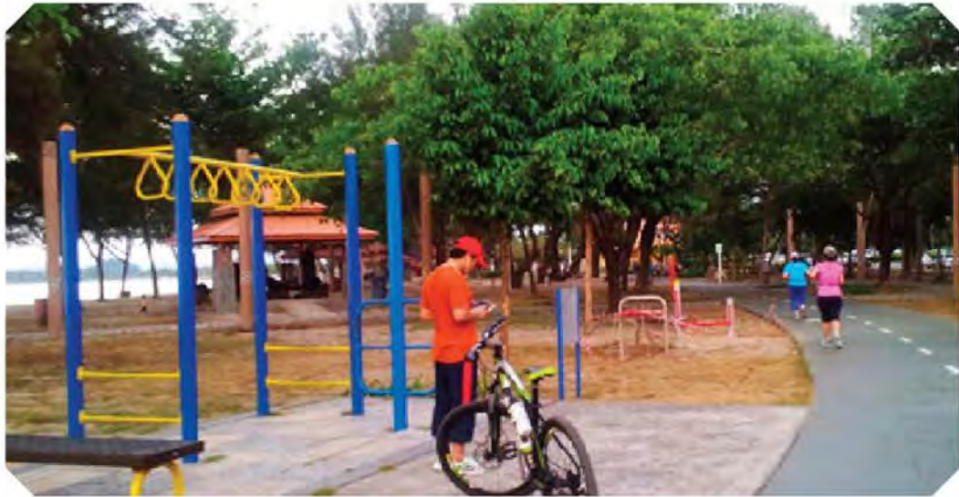
Completed Cycleway and Pedestrian Walkway at Tanjung Lipat, Kota Kinabalu
